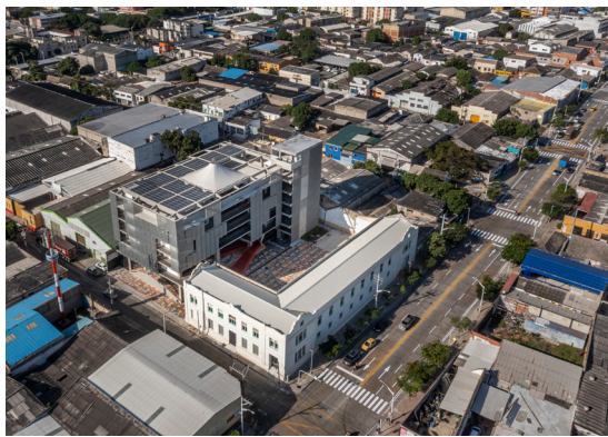
Aerial view of the public plaza
