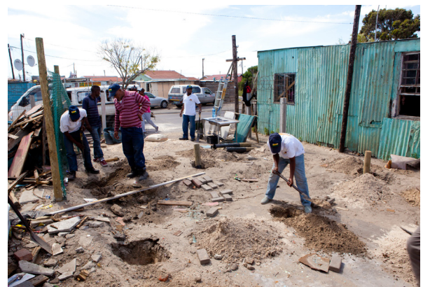
Building the first Empower Shack prototyp, Kayalitsha
