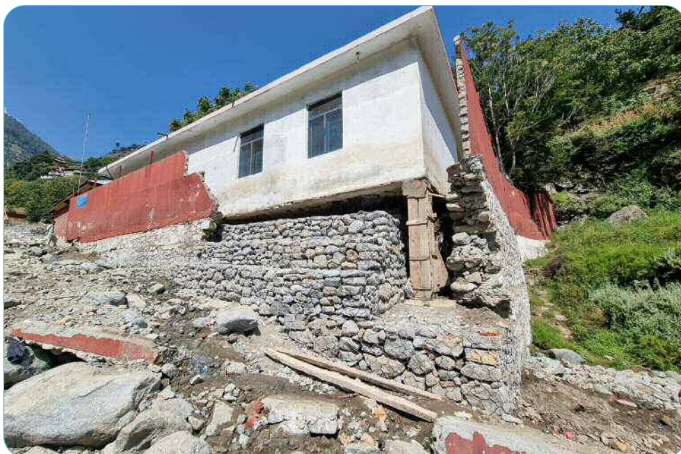
Fig. 07: Torwal school in the Swat Valley, Pakistan. Rehabilitation works with gabion walls. Christian Neuhaus, SDC 2022.
