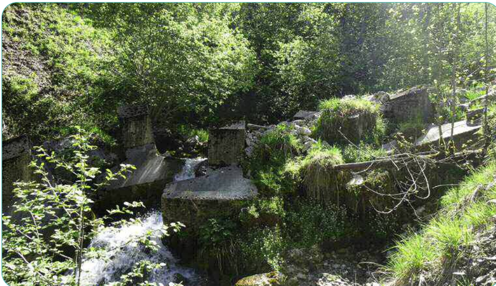
Fig. 06: Example in a small creek in Switzerland. Eric Bardou, UNHCR 2022.
