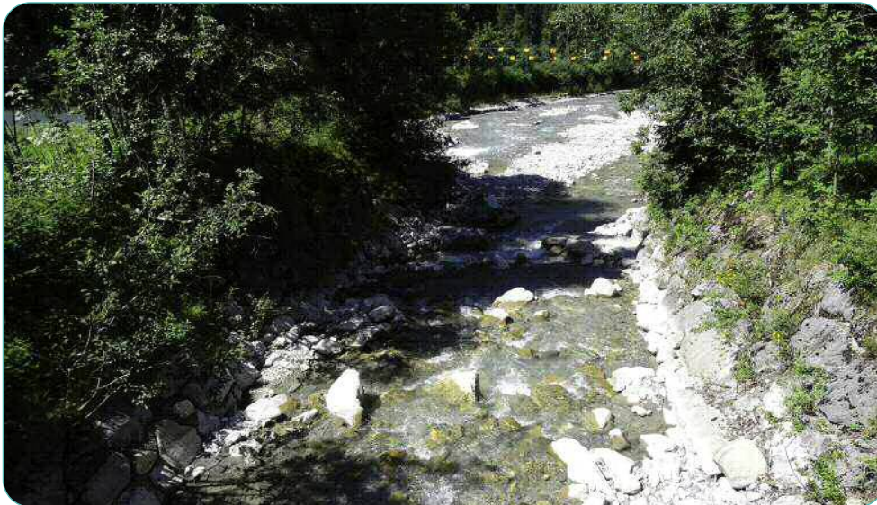
Fig. 05: Well-designed riprap can help shrub vegetation to grow (Big trees can cause riprap to collapse and must be removed). Eric Bardou, UNHCR 2022.
